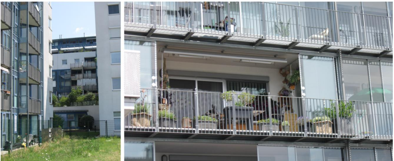
Figure.7. Internal balconies of residential buildings. Austria. (author's photo)
