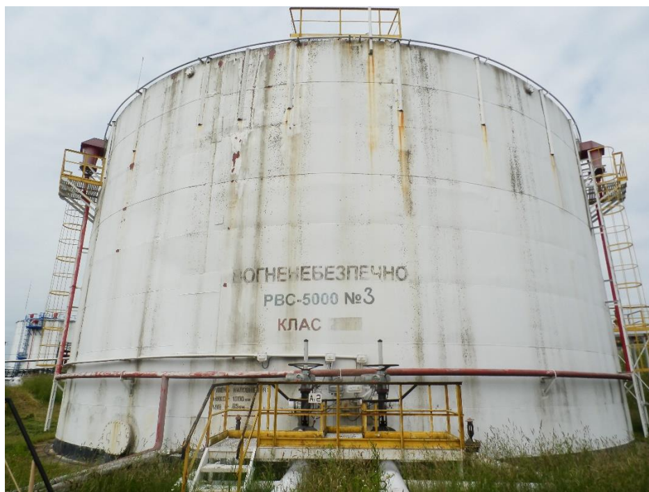
Fig.. 1. Steel tank, 5000 m 3 . General view.
