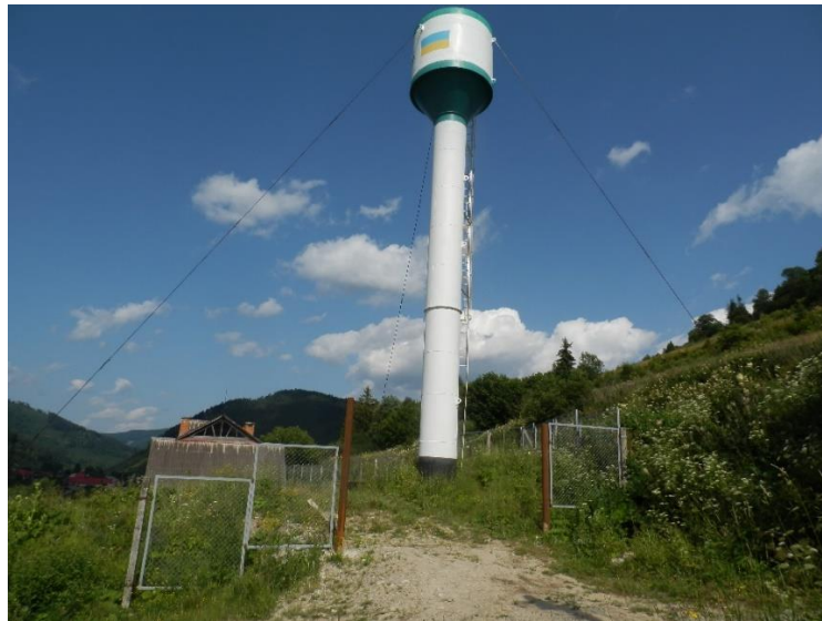
Fig.. 3. General view of the water tower.
