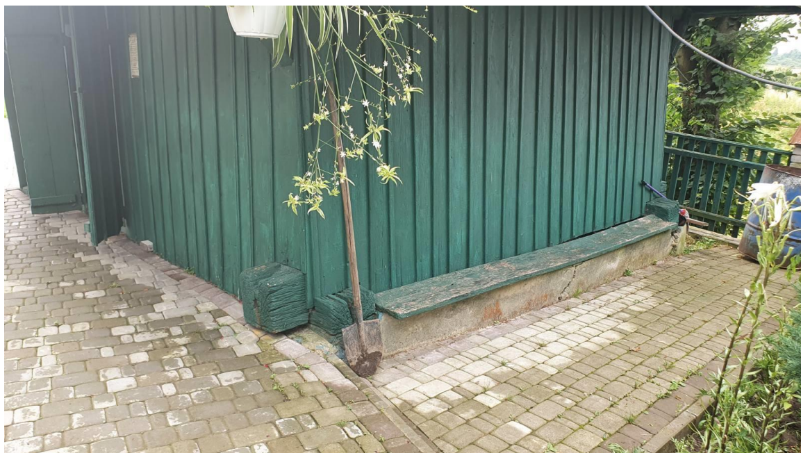
Figure 2. View of support beds and beams
