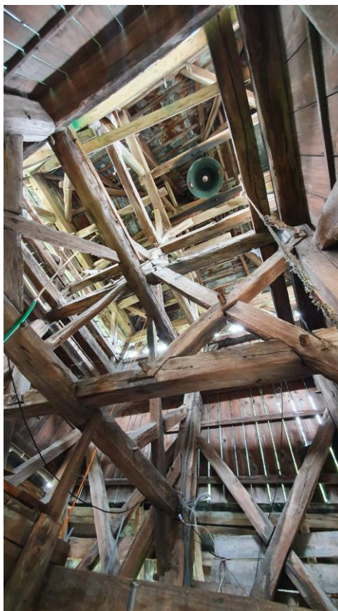
Figure 3. General view of structures from the inside
