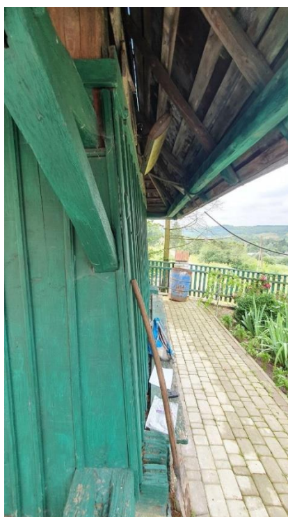
Figure 4. View of the inclined side wall
