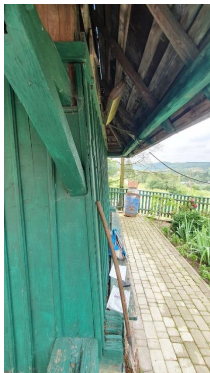
Figure 4. View of the inclined side wall
