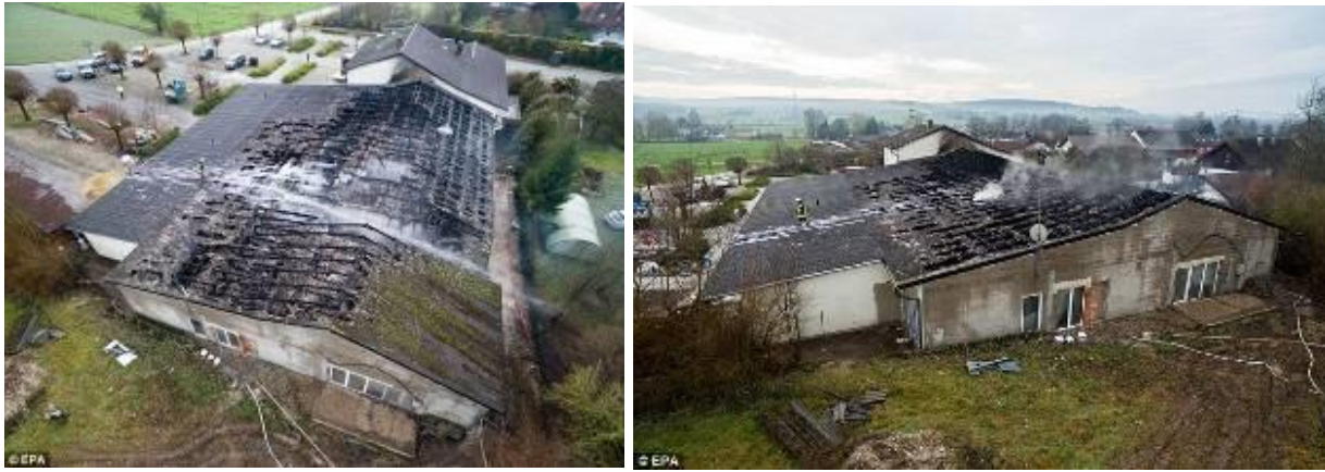
Fig.3. Fire destroyed a shelter for migrants in Rossbah [15]
