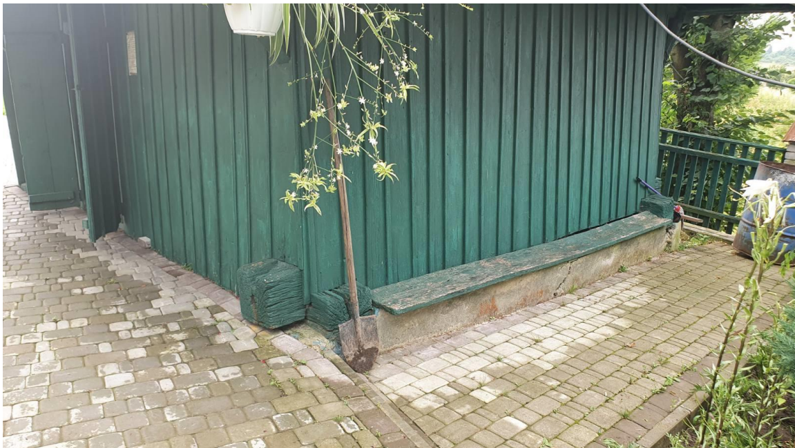
Figure 2. View of support beds and beams
