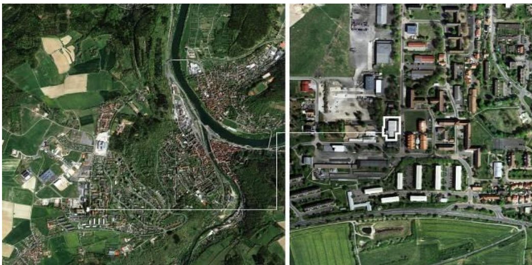
Fig.6. Arrangement of housing for workers in the structure of the city. Wertheim (coordinates: 49.753339 "N 9.495902" E)
