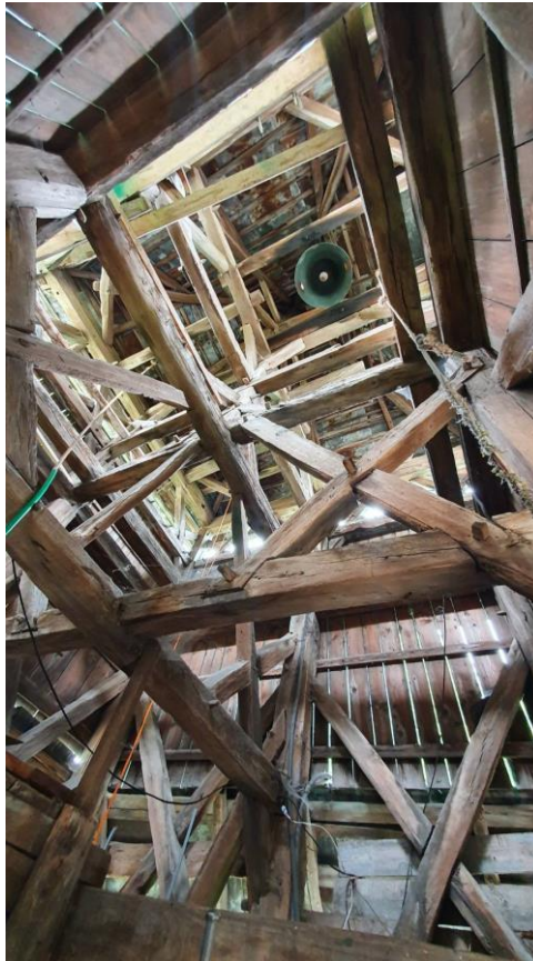
Figure 3. General view of structures from the inside
