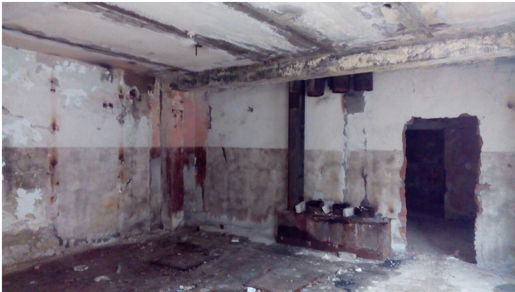
Figure 4. View of the room in axes "8-9/A-B"
