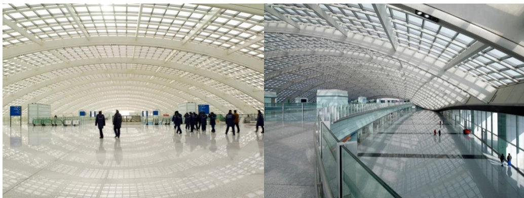
Figure 3. General view of structures and interior
