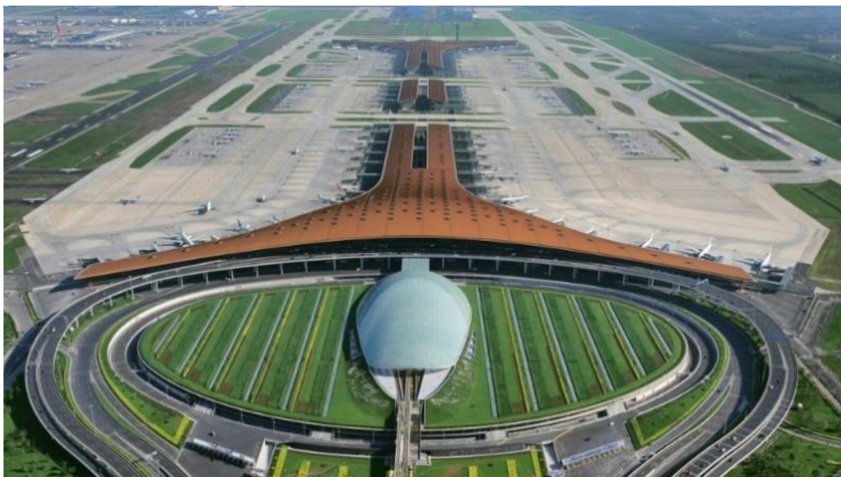
Figure 1. Bird flight view of the building
