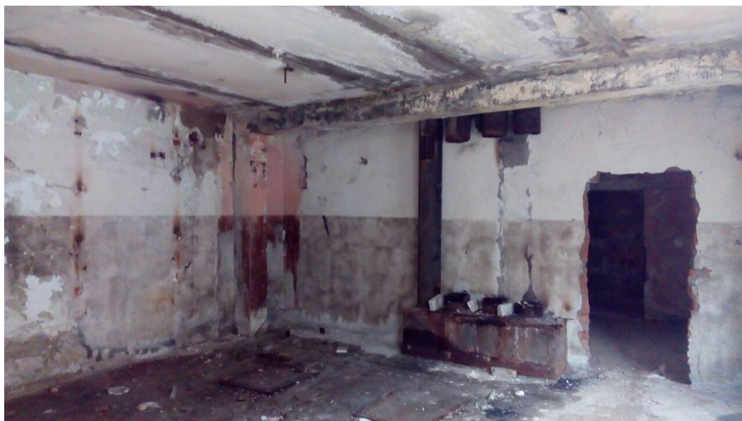
Figure 4. View of the room in axes "8-9/A-B"
