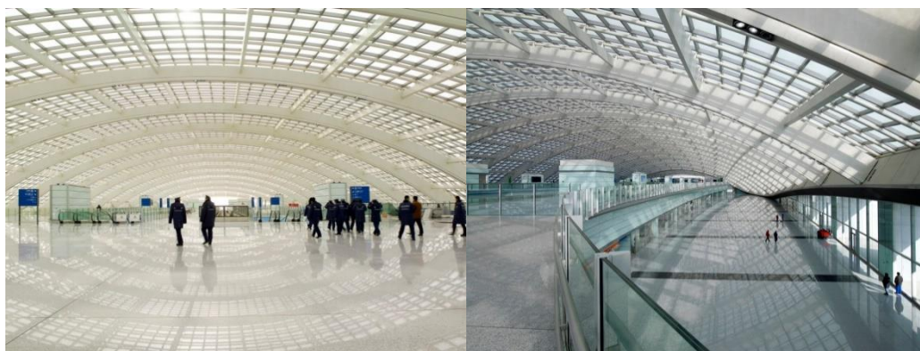
Figure 3. General view of structures and interior
