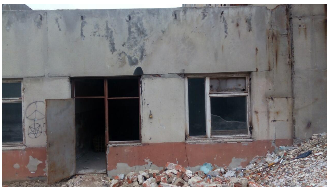
Figure 5. View of the facades of the existing building along axis "A" in axes "8-10"
