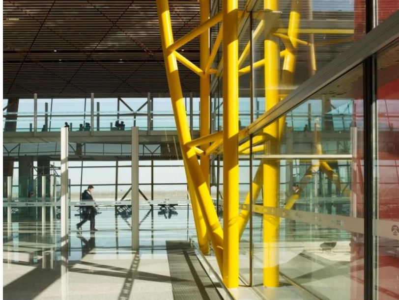
Figure 4. Supporting steel trusses
