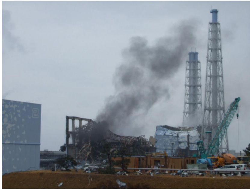
Figure 3. March 21, 2011, photo of damaged Unit 3 (middle) and Unit 4 (right) reactor buildings. Unit 2 is shown on the left margin of the photo ( http://photo.tepco.co.jp/en/date/2011/201103-e/110321-01e.html ) [2].
