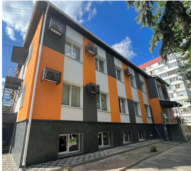
Figure 1. Completion of the implementation of energy-saving measures in the administration building in Vyskhorod, Kiev region.
