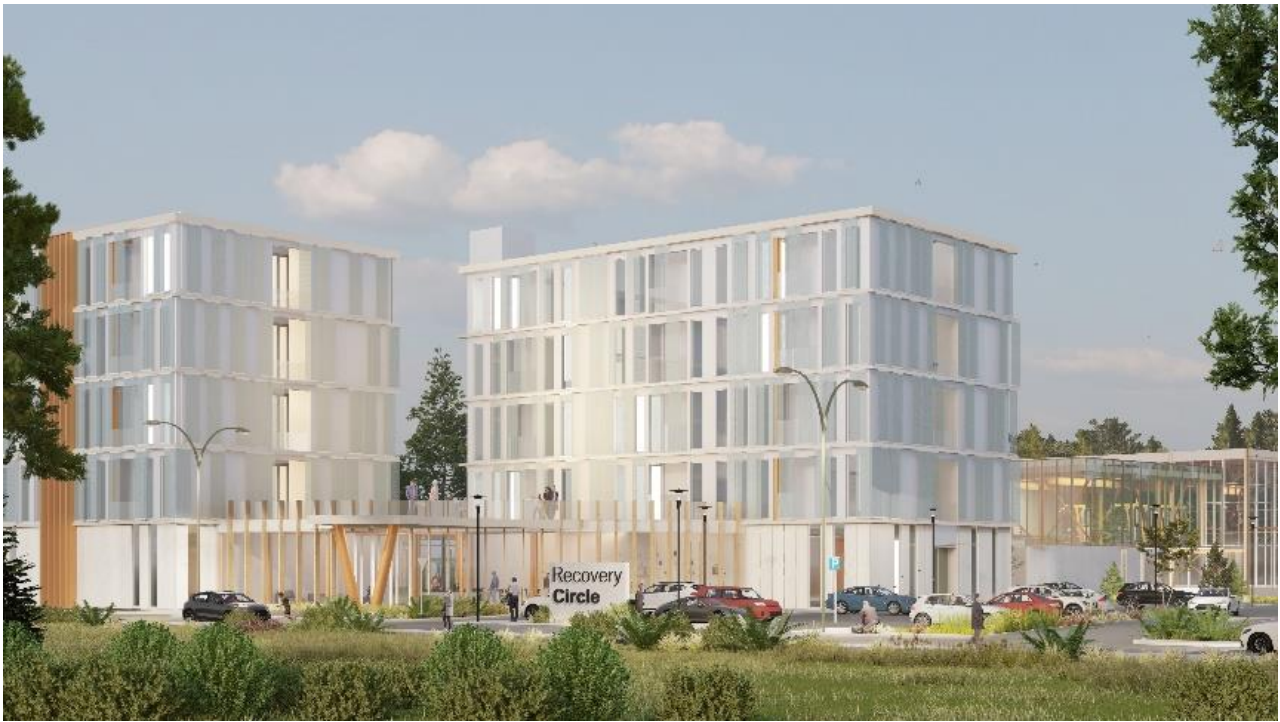
Figure 7. General view of the building
