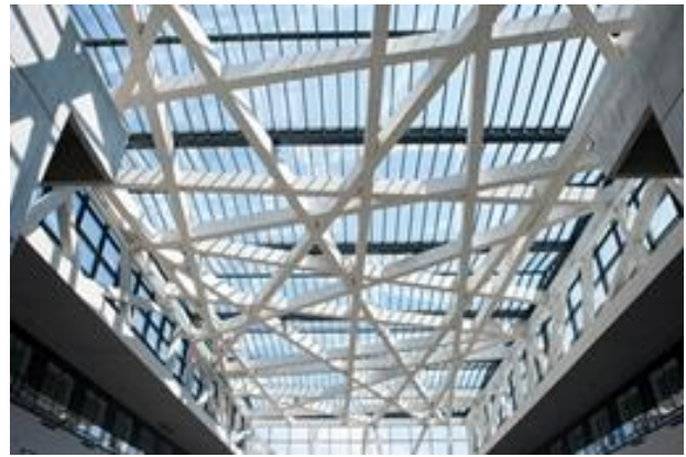
Figure 4. Atrium roof structure
