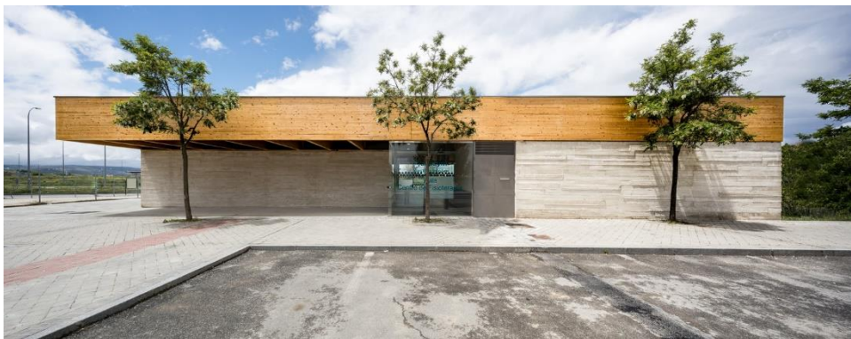
Figure 3: exterior of the medical center
