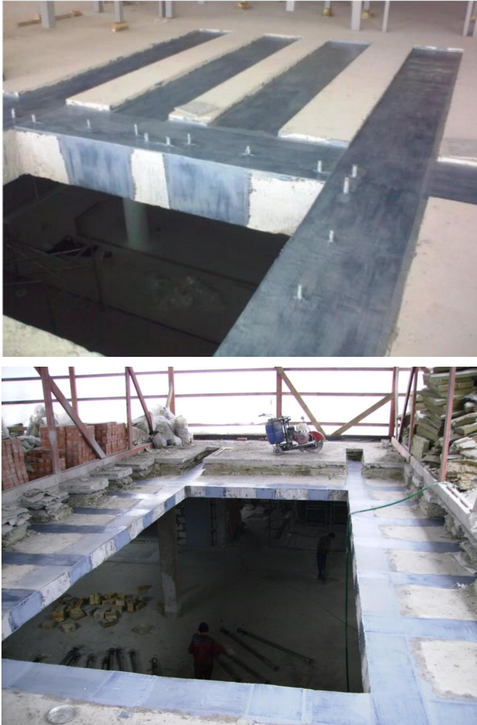
Figure 5. Examples of the use of carbon composite materials in the arrangement of holes
