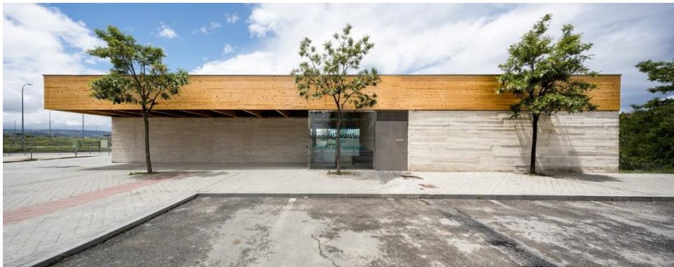
Figure 3: exterior of the medical center
