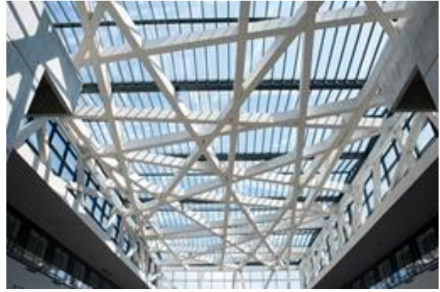
Figure 4. Atrium roof structure
