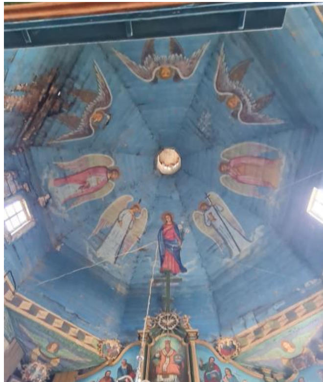
Figure 6. Photo of the dome from the inside
