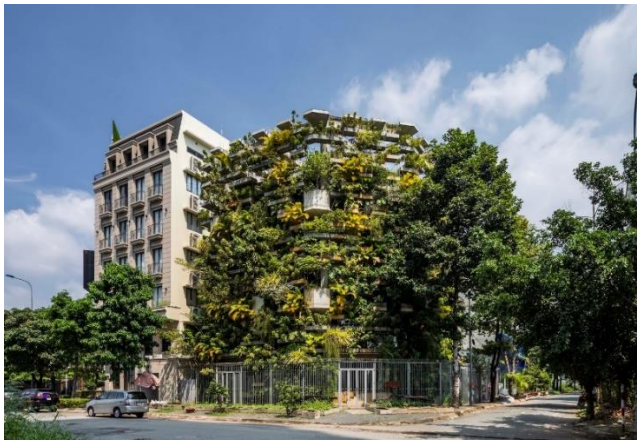
Figure 13. Adding green facade to the existing landscaping of the office building in Ho Chi Minh City, Vietnam (Abdel H., 2023)
