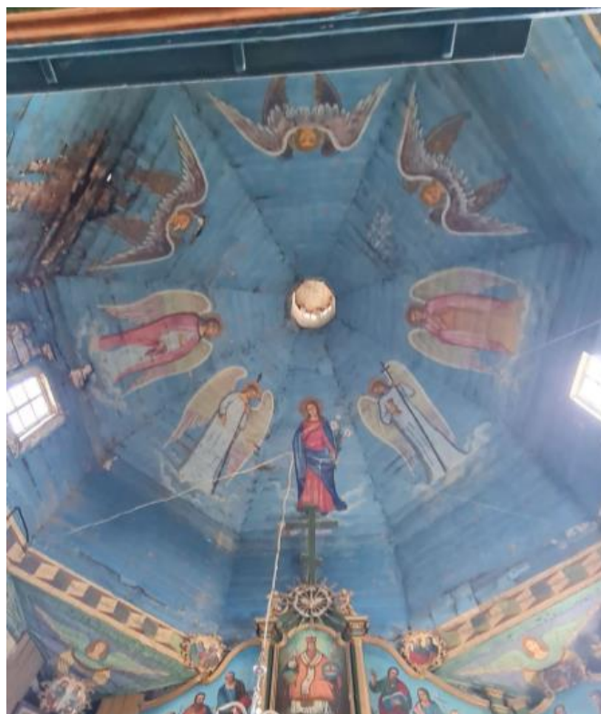
Figure 6. Photo of the dome from the inside
