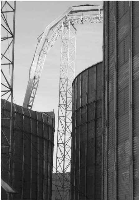
Figure 6. Lattice vertical rack between silos #4 and #6 and continuous lattice truss of the conveyor gallery
