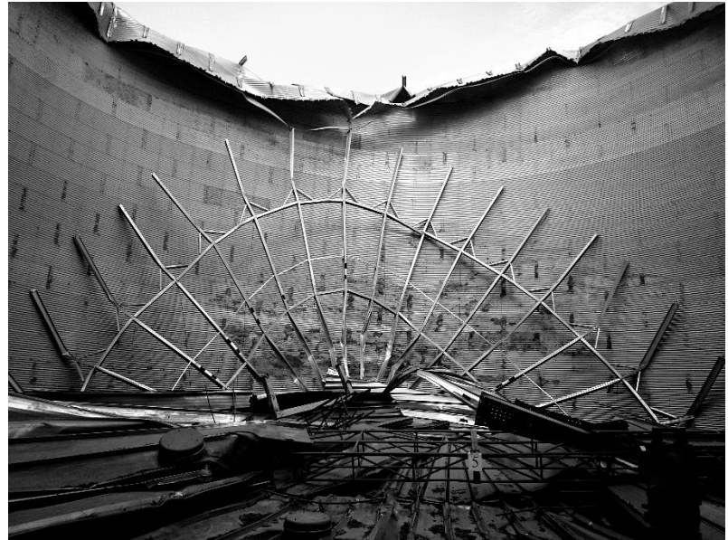
Figure 7. Hanging of the destroyed elements of the load-bearing structures of the conical coverings of silo #5 on the contour of its wall
