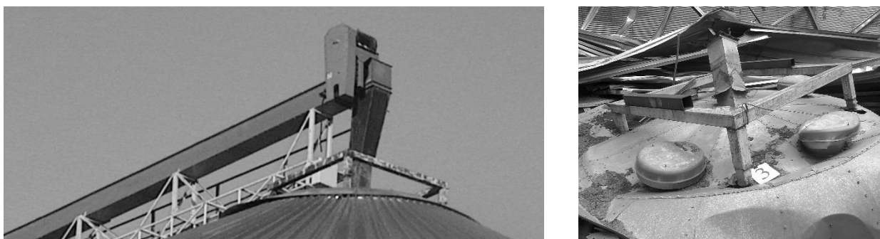
Figure 5. Rigid fastening of the lattice trusses of the conveyor galleries above the silos through the "chair" to the central ring of the conical cover
