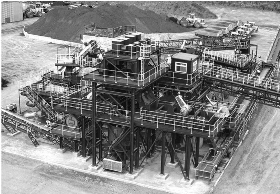
Figure 4. Processing Plant in Langton (Great Britain)
