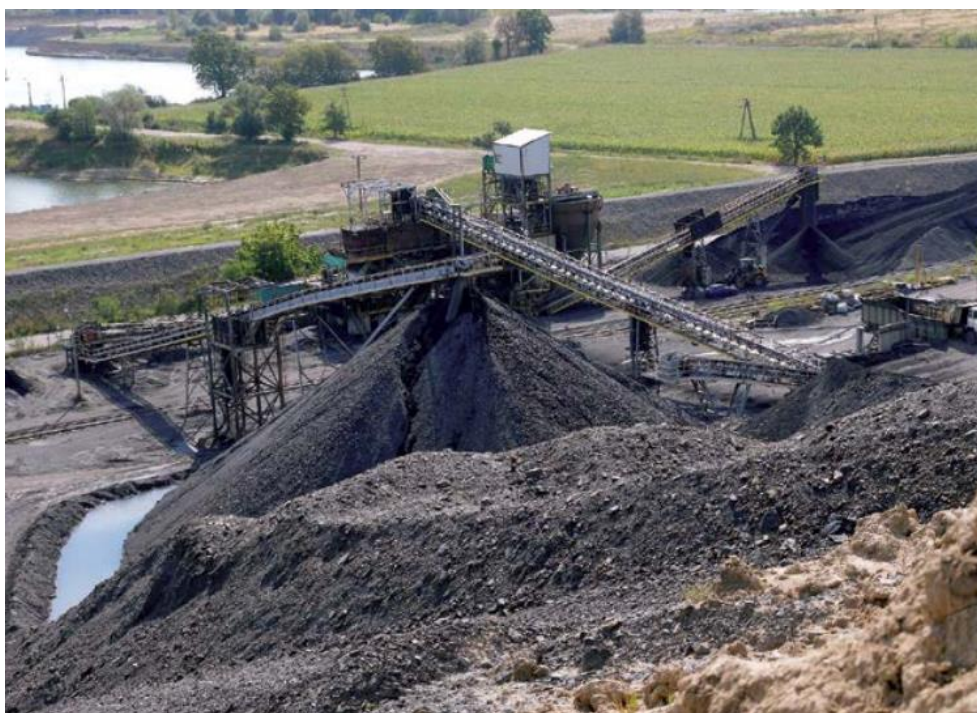
Figure 3. Coal plant in Buków (photo by Ł. Gawor)
