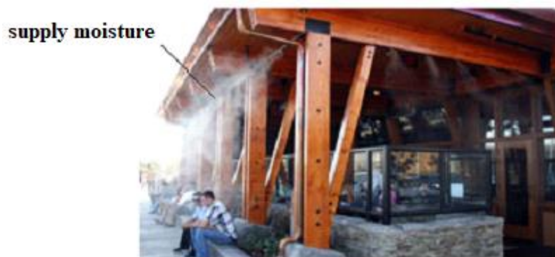
Figure 7. Application of humidifiers in working areas in the open area
