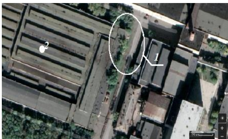
Figure 15. The territory of the rest area of the workers of the "Southern Machine-Building Plant" (Google Earth Image, 2024): 1 – summer cafe, 2 – foundry [518]
