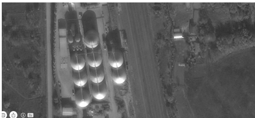
Figure 1. Aerial photography of the territory of the enterprise in the Khmelnytskyi region, before the destruction of the silos (photo from Google maps)
