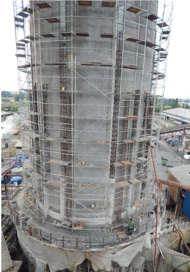
Figure 7. In the process of performing amplification
