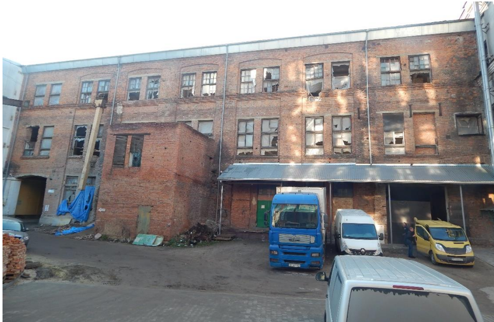
Figure 9. General appearance of the facade of the building during the survey
