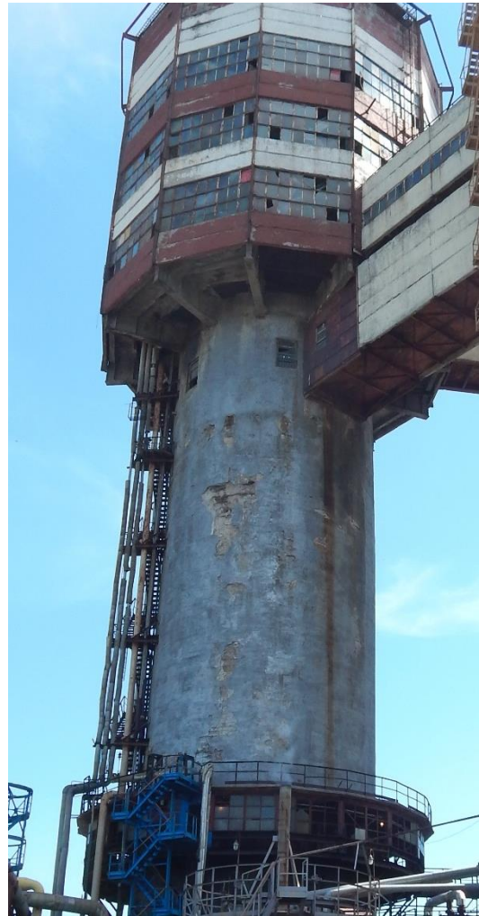
Figure 5. General view of the tower before reinforcement
