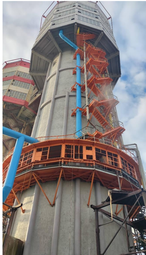
Figure 8. General appearance of the tower after strengthening and repair
