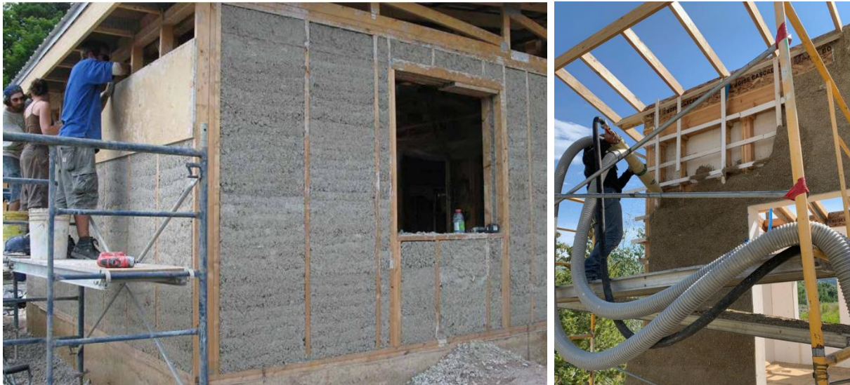
Figure. 1. Using hemp concrete by mixing at a construction site for the construction of wall structures
