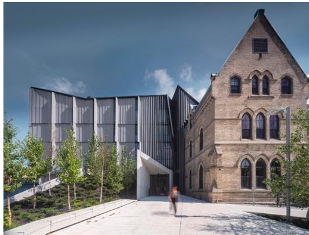
Fig. 4. General view of the historic building with modern extension
