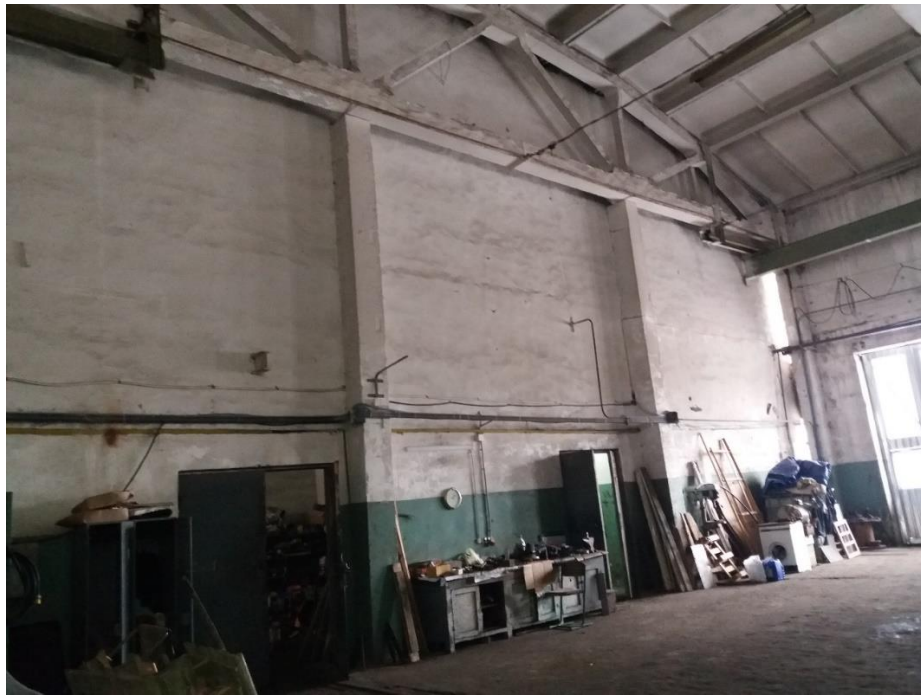
Figure 4. Photo of the existing interior of the building [made by the authors]
