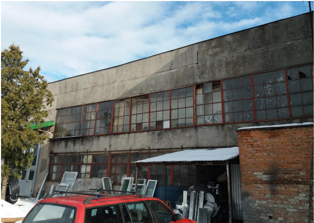
Figure 3. Existing building facade before reconstruction [made by the authors]
