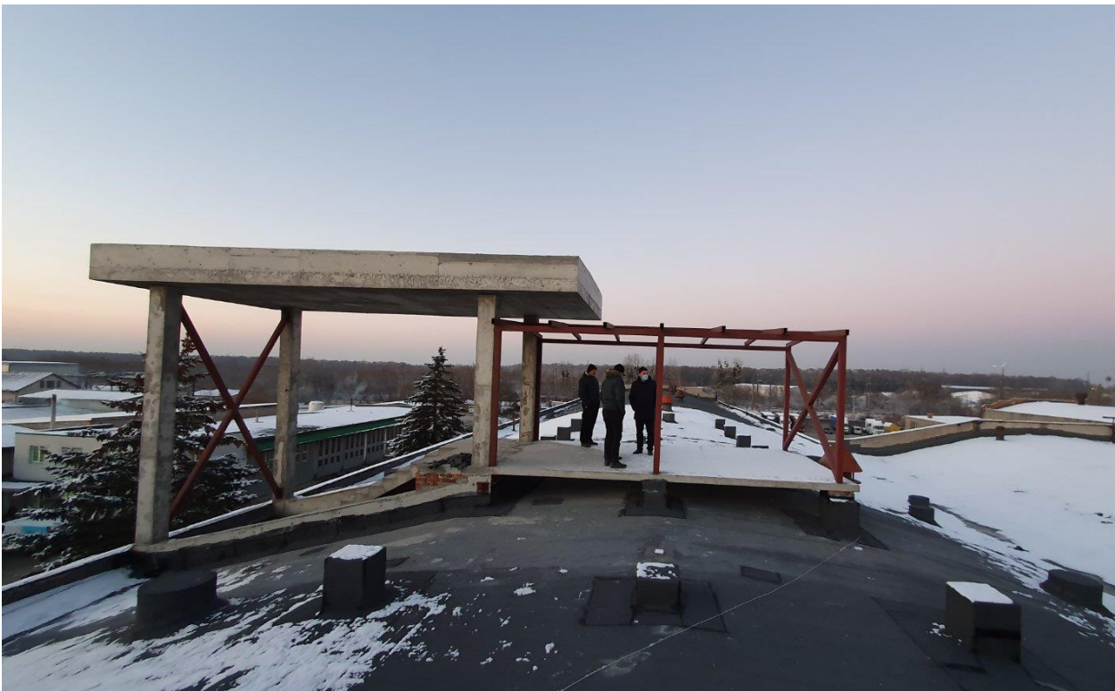
Figure 9. Roof at the terrace location [made by the authors]
