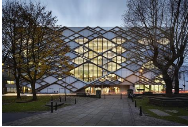
Fig. 2. Main façade of The Diamond [ https://www.ngbailey.com/case-study/45/the-diamond,-university-of-sheffield ]
